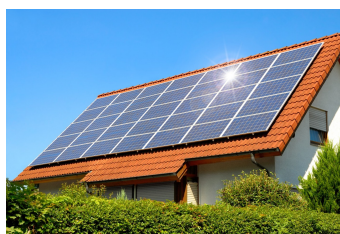
(b) Rooftop system [10]
